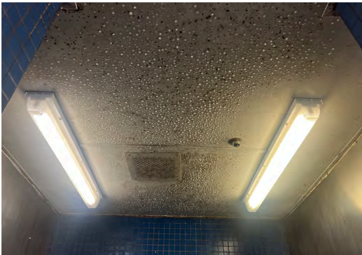
Bathroom ceiling exhibiting mold growth and condensation at Hartford Correctional Center.
