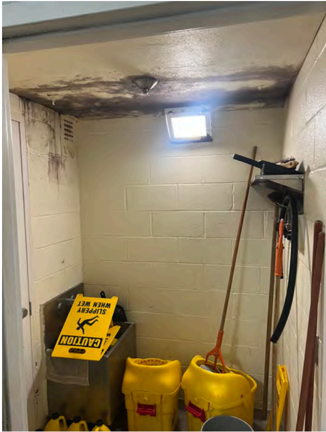
Mold-contaminated supply closet at Cheshire Correctional Institution.
