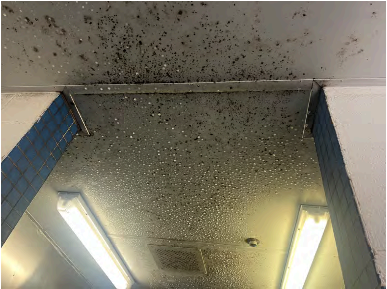
Bathroom ceiling with black mold and condensation at Hartford Correctional Center.
