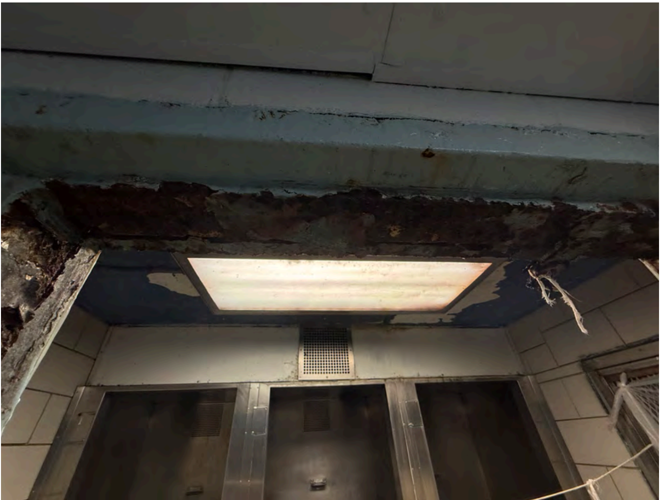
Shower door corroded with rust at Cheshire Correctional Institution.
