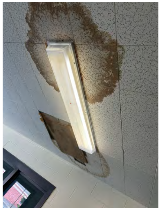
Water damage adjacent to a light fixture at Garner Correctional Institution.
