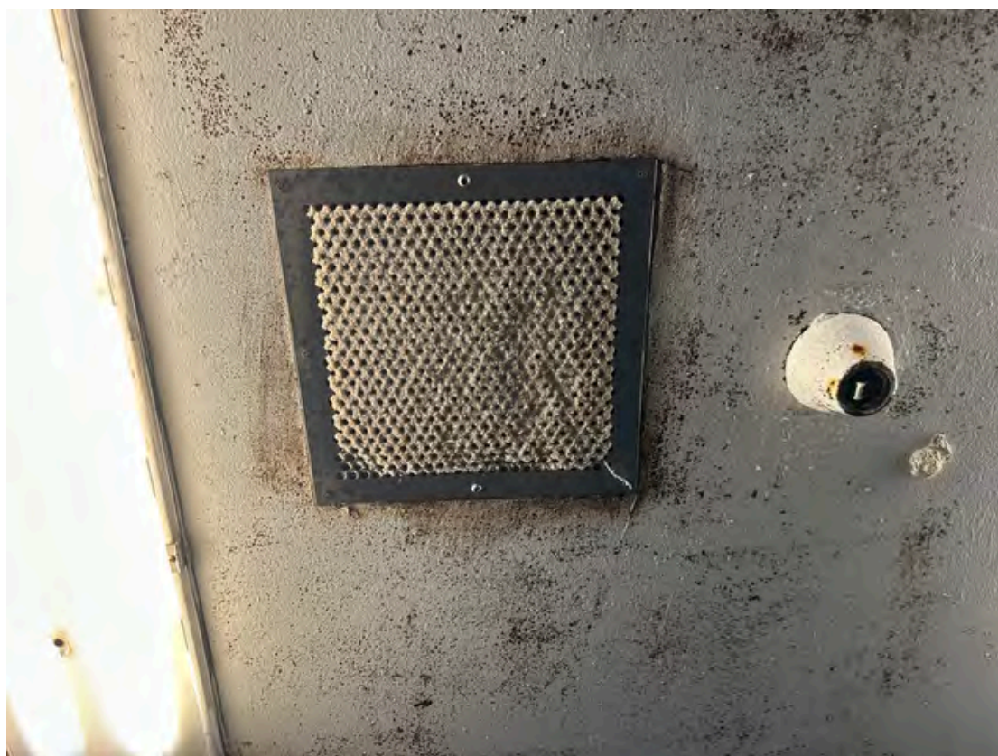
Mold present on a shower ventilation unit at Hartford Correctional Center.
